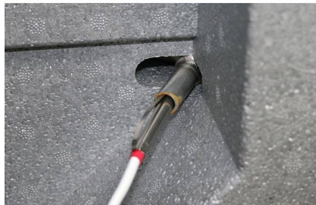
Figure 13: Clamping strap with temperature sensor of the hot water tank
